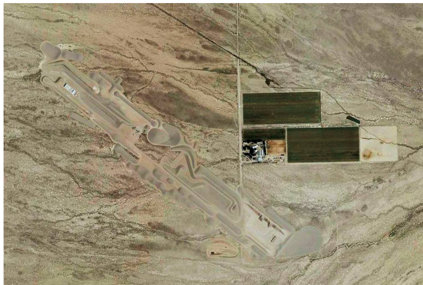
Aerial view of Heizer's 'City' under construction in Nevada
